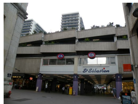
Hammerson's new shopping centre - they are planning to do it up!
