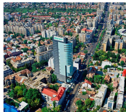
Globalworth's new tower in Bucharest
