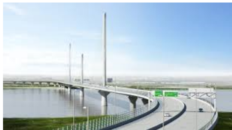
The Merseyside Gateway Bridge project
