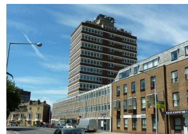
One of Empiric's student accommodation blocks
