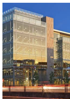
Green REIT's new office at One Albert Quay in Cork
