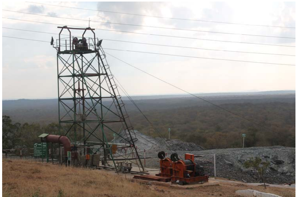
Figure 18: Exploration shaft at the GG prospect in June 2016
