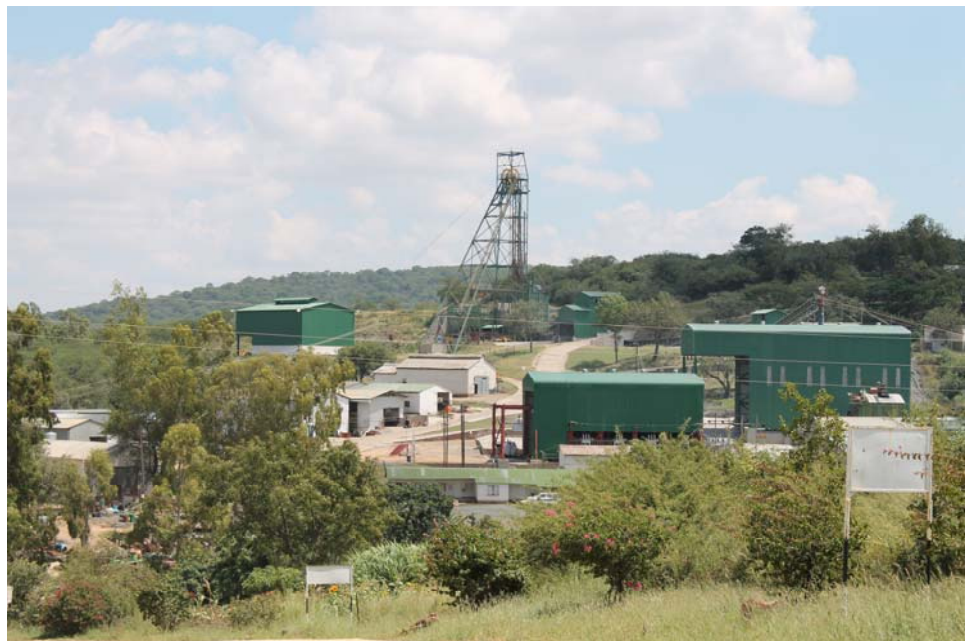
Figure 8: No 4 Shaft and plant at Blanket mine as at March 2013
