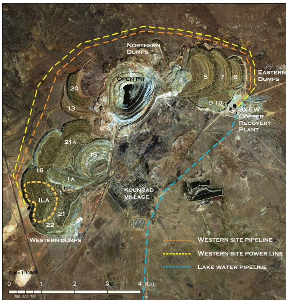
Figure 19: Aerial view of the dumps
