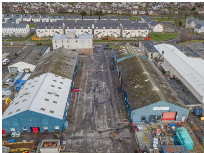
Figure 4: Burnside Industrial Estate, Aberdeen - exterior
