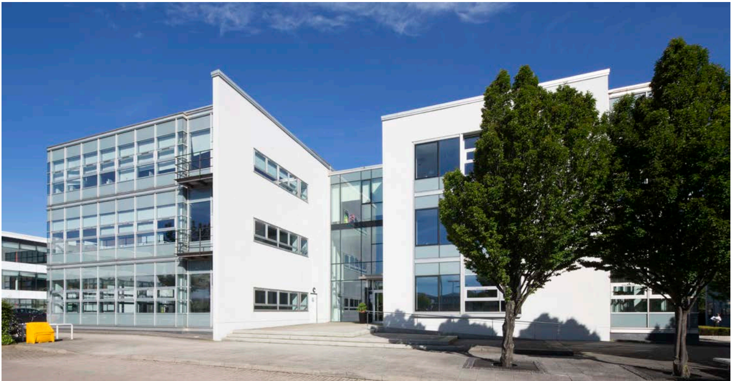
Figure 1: 3 Lochside Way, Edinburgh – exterior
