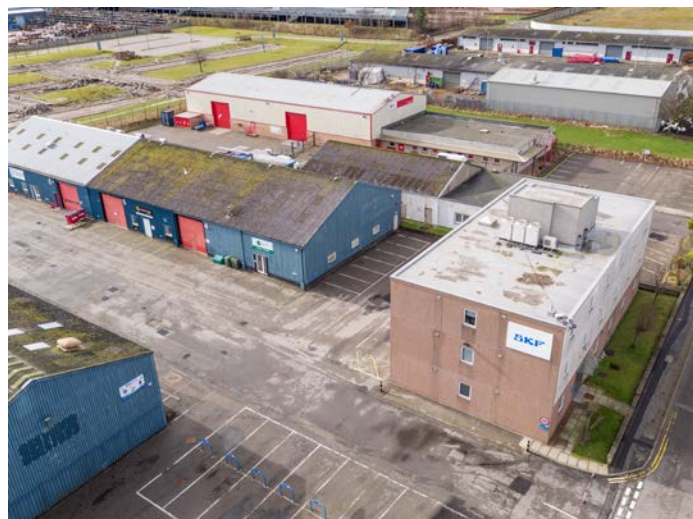
Figure 5: Burnside Industrial Estate, Aberdeen - exterior
