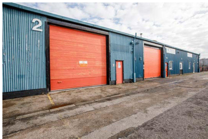
Figure 7: Burnside Industrial Estate, Aberdeen - exterior
