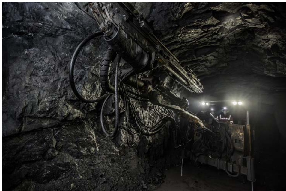
Figure 27: Jumbo drilling underground at Sasa
