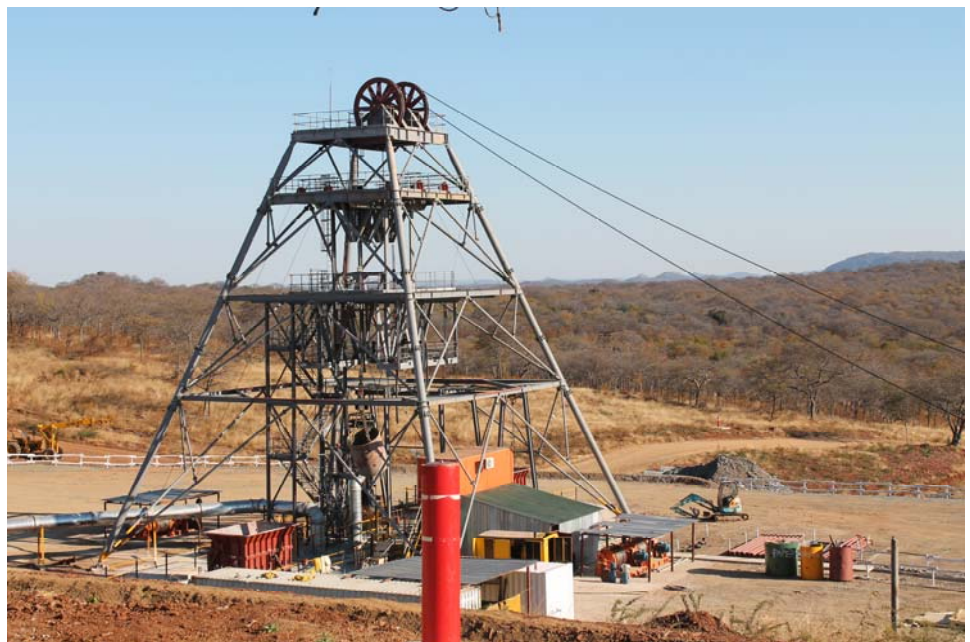
Figure 15: Headgear of the Central Shaft
