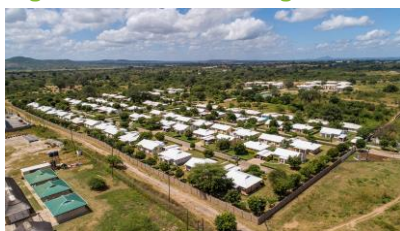
Figure 10: VDE Housing Estate
