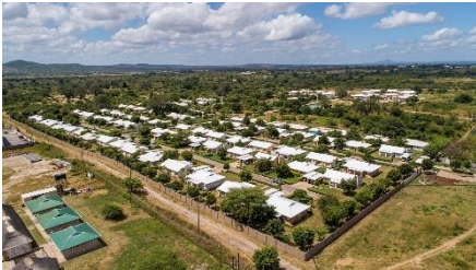
Figure 12: VDE Housing Estate
