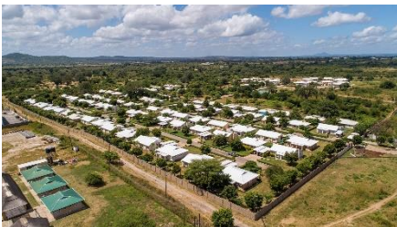
Figure 7: VDE Housing Estate
